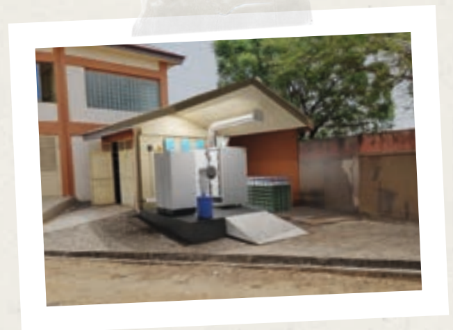
↳ Realisation concept for a hydrogen generation and storage unit powered by solar energy with a 20kW PEM electrolyser and a 10kW fuel cell
