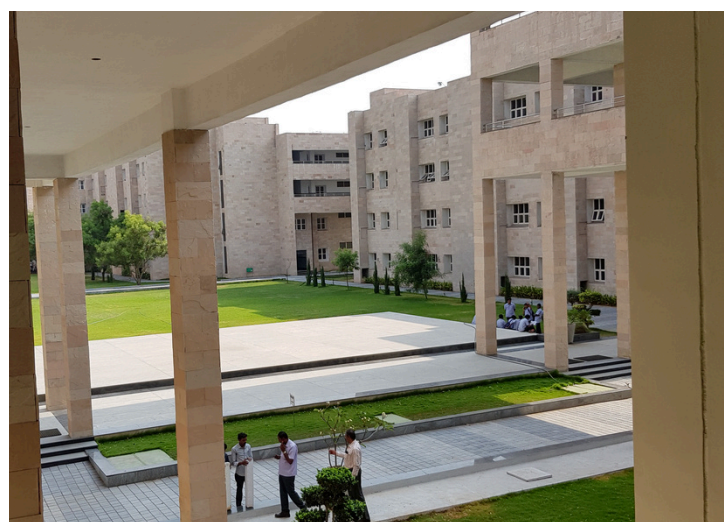
Figure 6: The new campus of the PSG College of Technology, India
