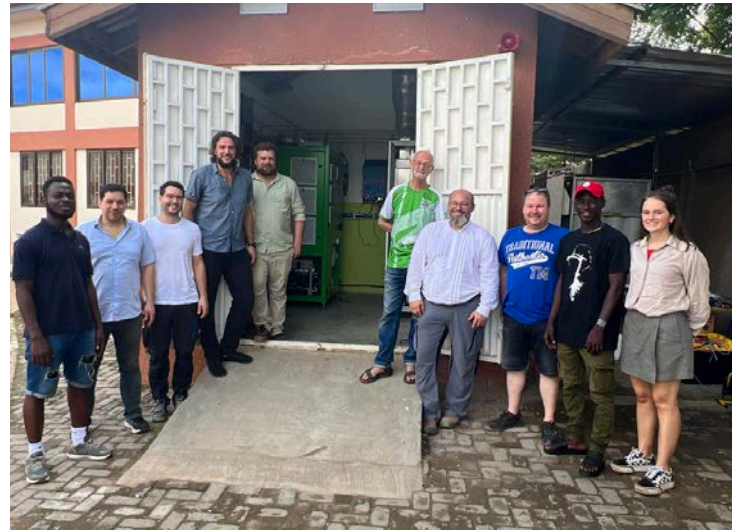
Figure 27: Green hydrogen for Ghana: The GH2GH team installs the first decentralised system for hydrogen production and reconversion in Tema (October 2024)
